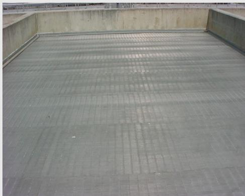
**The simple dewatering operation** is provided compliments of gravity, so the process costs practically nothing to operate. The low pressure process uses less polymer and energy. Manpower requirements is less than other systems, freeing your personnel to perform other important tasks, since the system practically runs itself — just turn it on, fill the bed, and turn it off!
